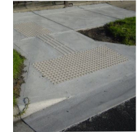
6 New Accessible Ramp
