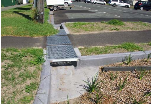
GRATED CONCRETE CHANNEL
