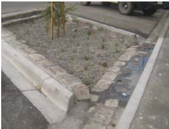
BLUESTONE PITCHERS WITH CROSS-FALL INLET
