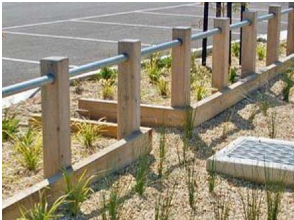
GALVANISED RAIL FENCE
