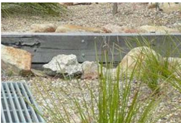
TIMBER RETAINING WALL TREATMENT
