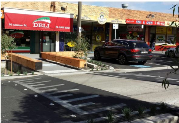
White herringbone pattern stencilled concrete
