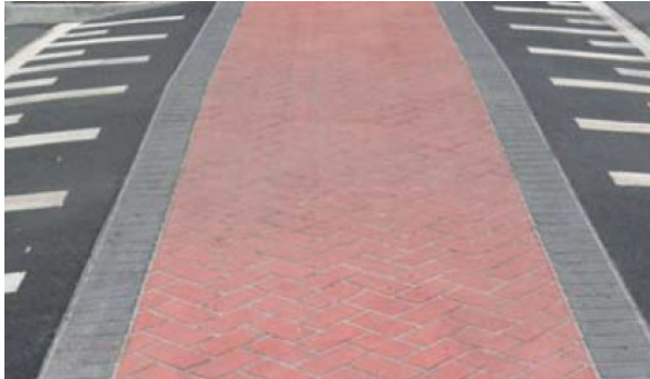
Red herringbone pattern stencilled concrete with grey edges
