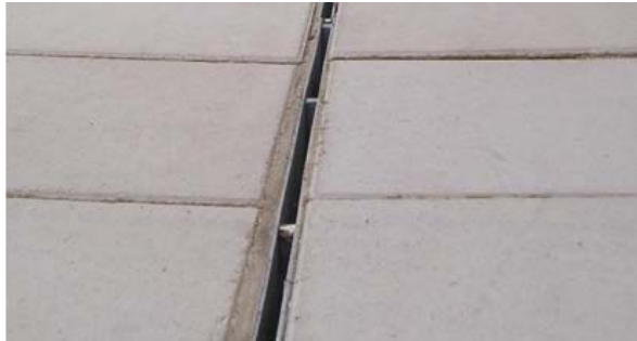
Brickslot for poured concrete or concrete pavers
