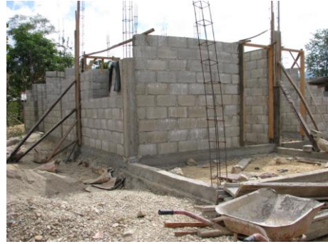
New maternity ward being built at the Aileu District Health Clinic
