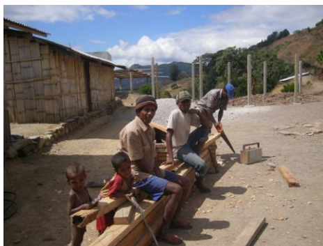
Carpenters constructing roof trusses for new classrooms at Teblor 'filial' school
