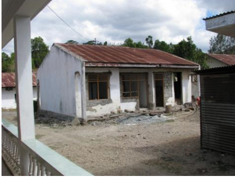
Renovations under way on midwives' accommodation in Aileu
