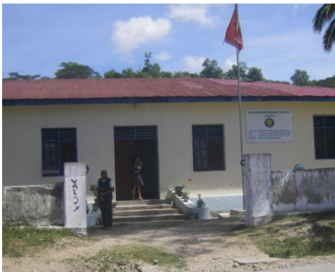
Temporary premises of ASTI
