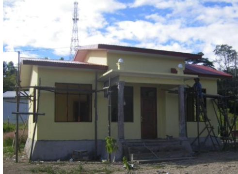
The new offices for the Aileu District planning staff
