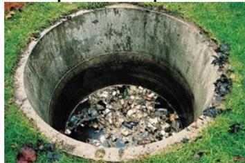
Gross pollutant traps (GPTs) are structures that use physical processes to trap solid waste such as litter. They are commonly used upstream of other treatment systems which remove finer particles.
