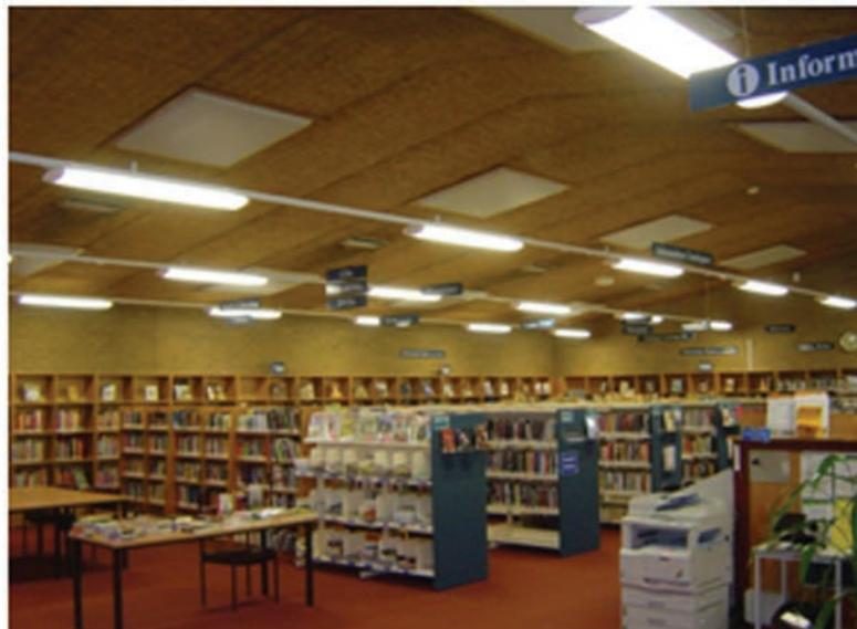
Before (left) and after (right) showing the improvement with the new fittings. The old T8 fluorescent light fittings remain because the polycarbonate covers act as an isolative barrier and the cost of removing and reinstating the ceiling lining could not be justified. It was easier and simpler just to leave the old fixture where they were and hang new fittings underneath the ceiling.
